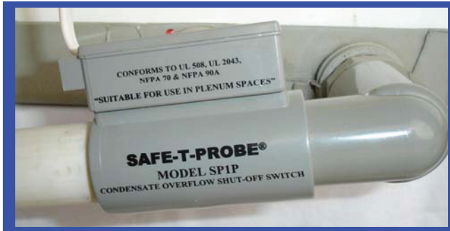
INLINE (PRIMARY DRAIN) INSTALLATION
