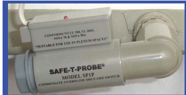
PLUGGED (AUXILIARY DRAIN) INSTALLATION
